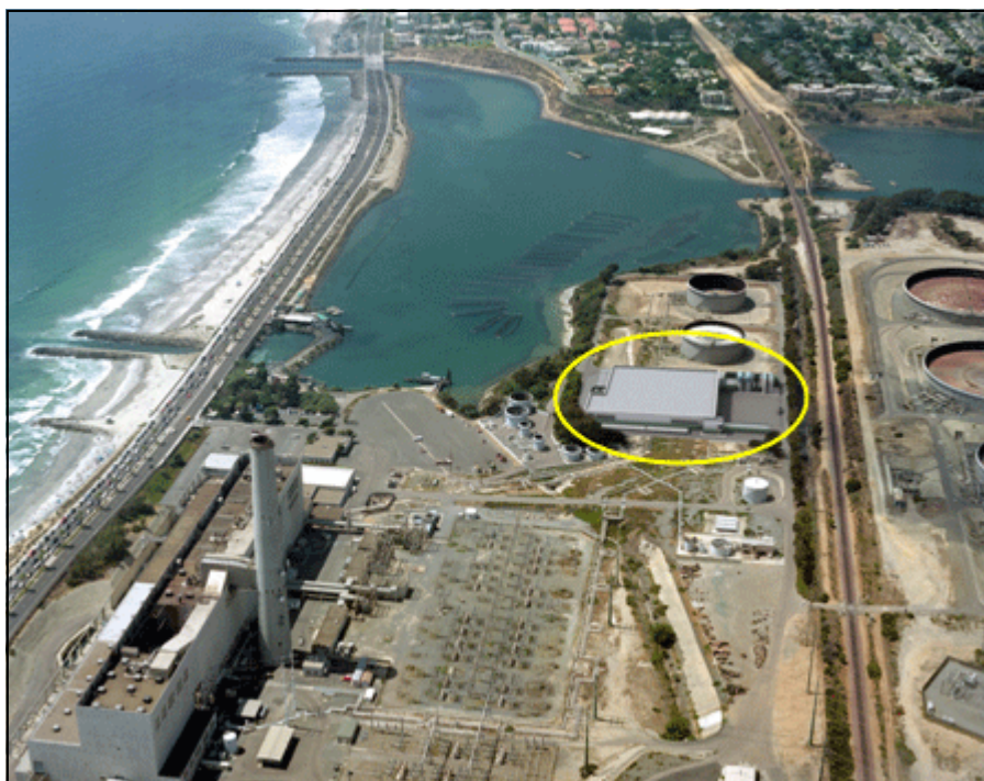
The Carlsbad Desalination Project, located at the Encina Power Station in the City of Carlsbad, consists of a 50 MGD (56,000 acre-feet per year (AFY)) seawater desalination plant and associated water delivery pipelines.
