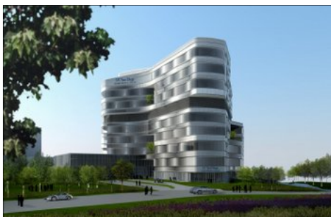
UCSD is planning to build the 245-bed Jacobs Medical Center next to Thornton Hospital in La Jolla
